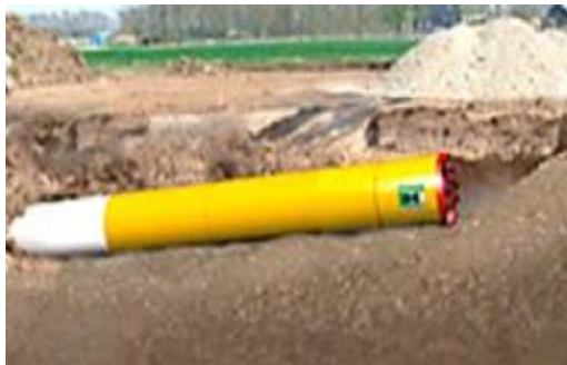
Plate 3.5: MTMB machine at exit location
