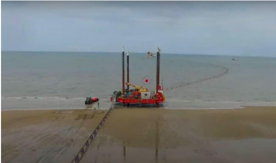
Plate 3.7: Example intermediate pulling platform barge
